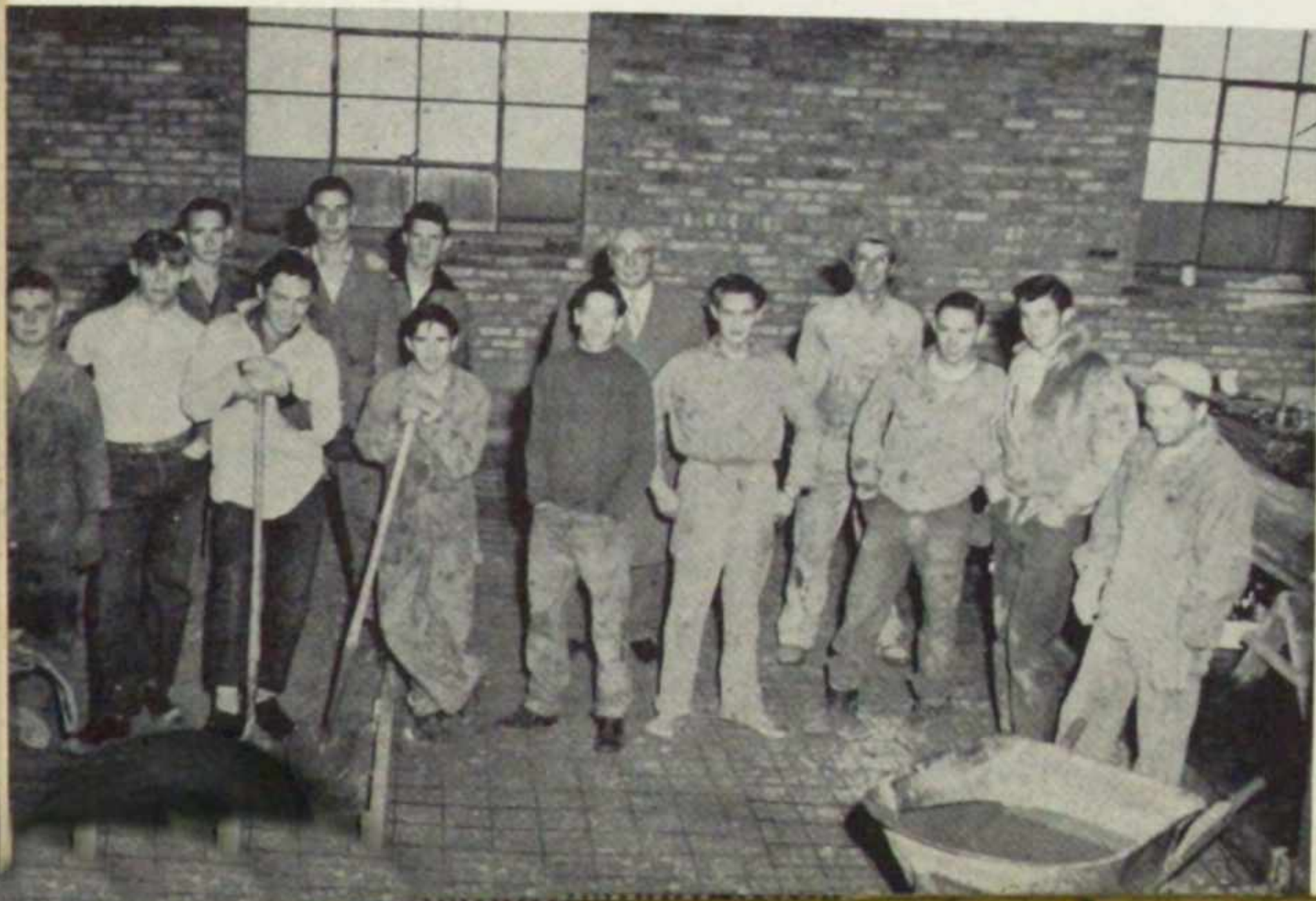
Boys who helped build the new T and I Building
